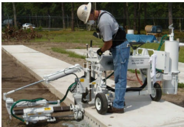
Worker drilling horizontal holes in concrete slab with a dowel drilling rig. The shroud surrounds the drill steel where it enters the concrete and the dust collector is the canister on the right. Worker is wearing respiratory protection.
