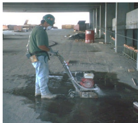
Worker using water to suppress dust while operating floor grinder.
